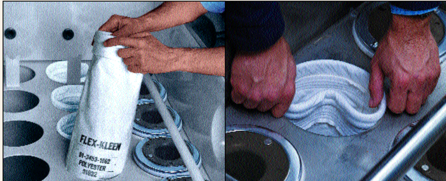
1. Insert the bag through the hole in the tube sheet.
